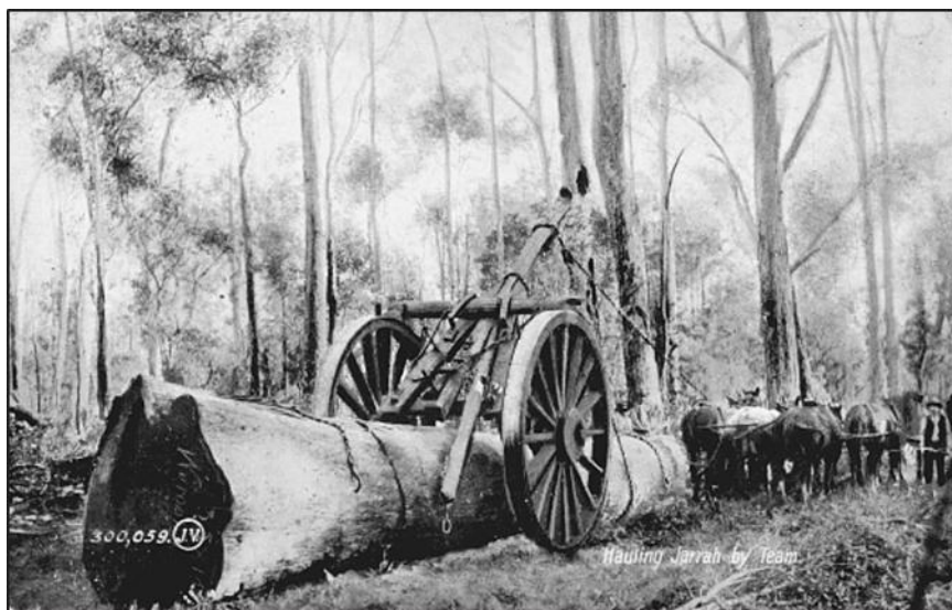
Log Transport - horse team pulling log using a whim - Wellington Mill area early 1900s
